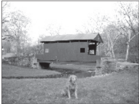
Hanging at Ebenezer Covered Bridge.
