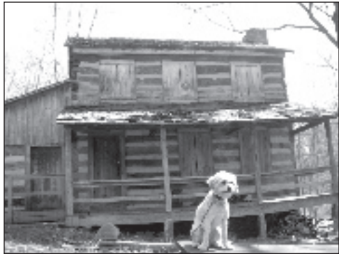
The Carpenter House would have been a formidable structure on the 1820s frontier.
