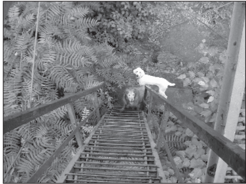
The open grate steps and open railings will keep your dog on the ground at the lookout tower atop Goat Peak.
