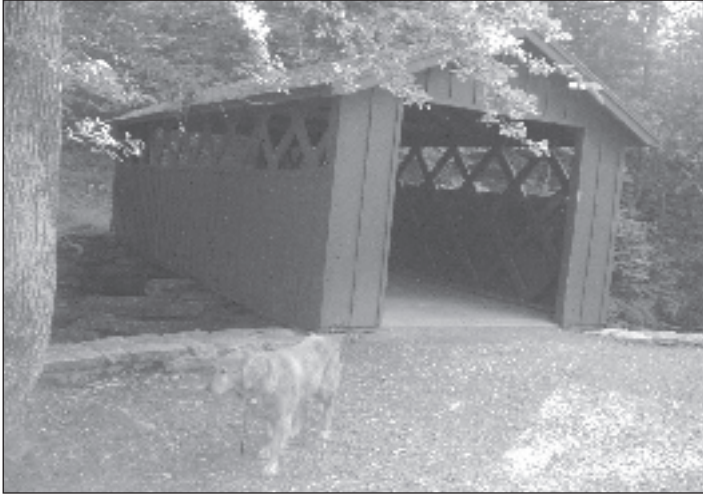
The open-latticed covered bridge in Chatfield Hollow.
